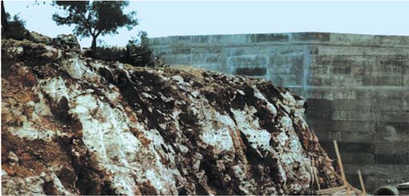
Photo 21 On the bridge: Road No. 447 / Under the bridge: the Iskaka-Salfit road
